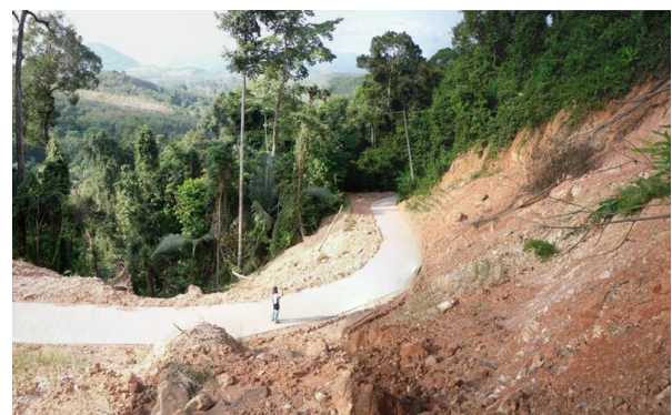
Fig. 7. Cut slope site in Kanjanadit, Suratthani.
